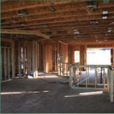
Construction in Progress
